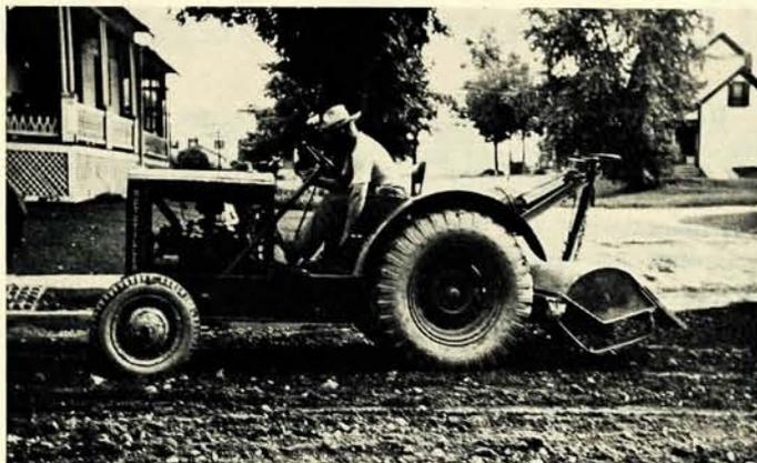
Above a Rototiller Tractor was used to make the concrete streets in Granville, NY, north of Troy. Below, Carl Kelsey himself waters a soil-cement driveway being constructed in the alley behind the Rototiller Factory, putting product-testing to practical use.
