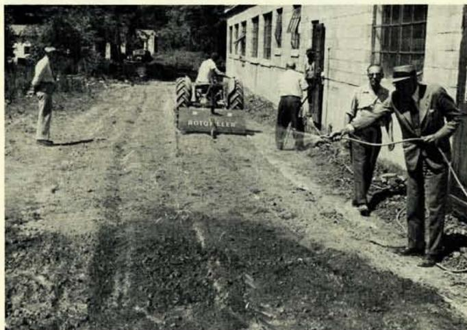
In 1937 Portland Cement acquired several of Kelsey's walking-model C-8 Rototillers for use in the process. They were found to be ideal for mixing cement with the soil and, in 1938, were used to lay 17 acres of concrete at the Golden Gate Exposition in San Francisco. When Portland Cement Company heard about Kelsey's larger tractor-drawn unit, they ordered a number of those for use in the construction of soil-cement runways at airports throughout the country.
