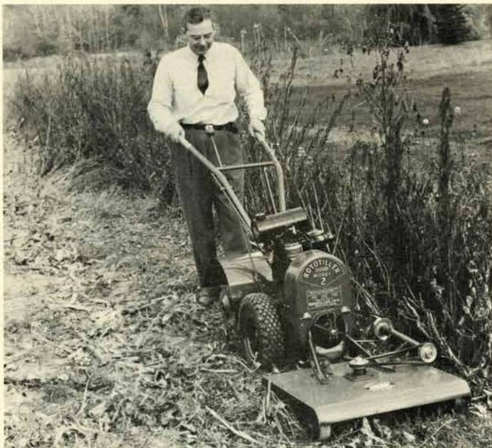
The Rototiller Model 2 was an improved version of the Model T. With its patented “Lightning Change Front”, many lawn and homestead accessories could be attached in just a minute or two. Here, Lyman Wood tries out the rotary mower attachment.
